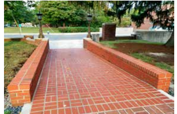
New Ramp from 2 nd Street to the "Park of the Valiant" honoring Electric Department.
