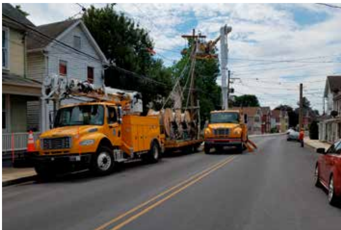
Pulling in New Conductor along Broad Street
