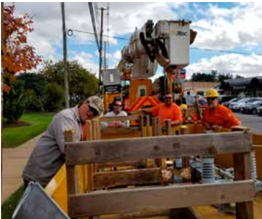
Line Crews Recap Repairs Made to a Damaged Overhead Switch
