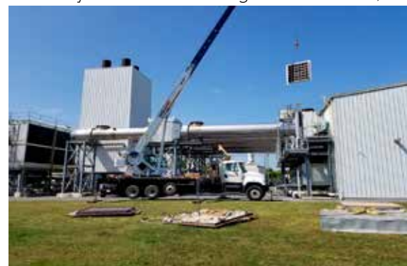
Replacing CO Panel at Orchard Park Generating Station
